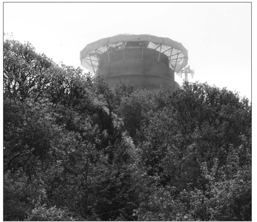
The mother ship has not landed, but a protective cover over the water tower on Edgemere Road does make it look a little otherworldly. Janis Hewitt
